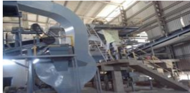
Unit 2 – SSP Granulation Plant
