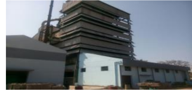
Unit 3 - New Reactive Dyes Plant
