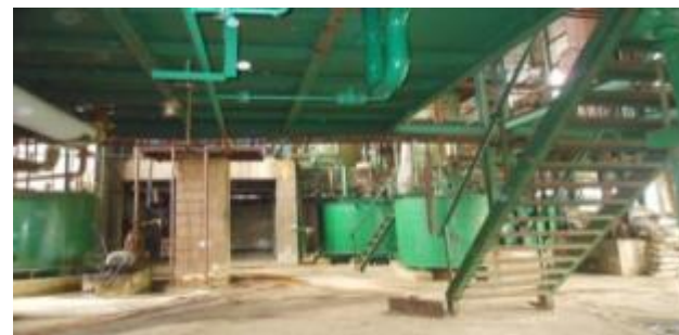
Sulphuric Acid Plant
